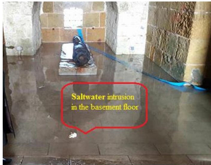
Fig (5): Saltwater intrusion inside the citadel.
